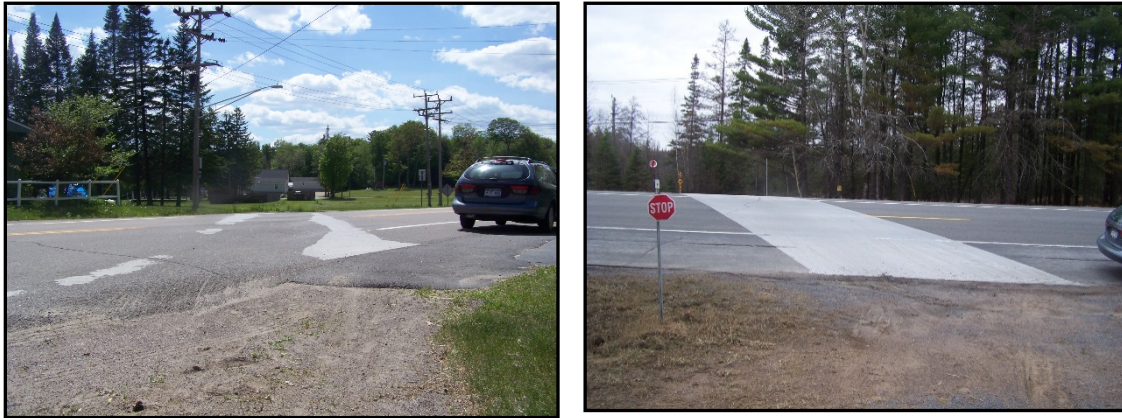
Figure 5.41 Thermoplastic Treatment for Snowmobile Crossing. The photo on the left shows a degraded treatment. The photo on the right shows an intact treatment.
