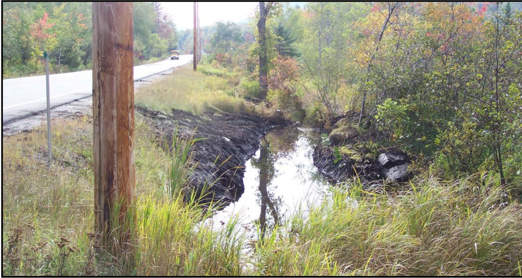
Figure 4.9 Ditching. Ditching is essential to manage highway runoff. But it requires a balanced approach to manage possible negative side-effects such as; impacts to water quality, movement of invasive species and the disposal of surplus material.
