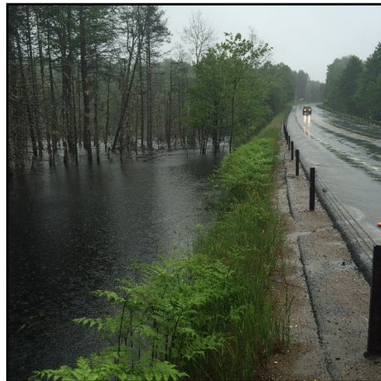
Figure 5.23 Beaver Culvert Impacts. Beavers have plugged a culvert forming a large water impoundment and creating a potential safety hazard.
