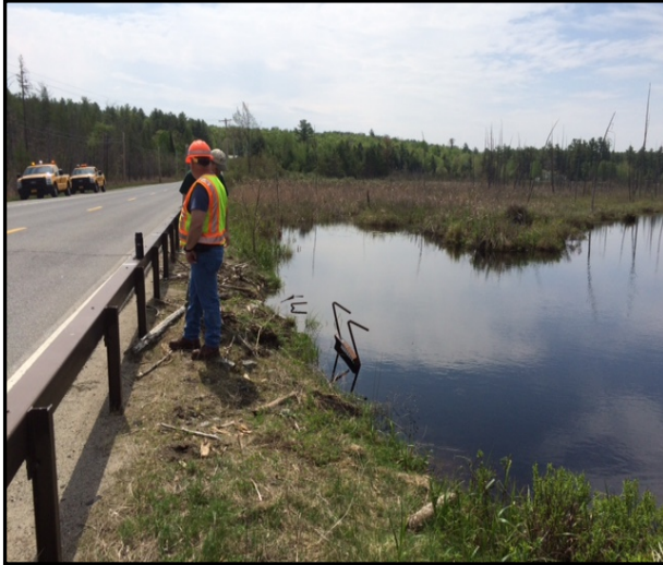
Figure 5.24 Beaver Impacts. Beaver complexes create high water which can impact the transportation infrastructure.
