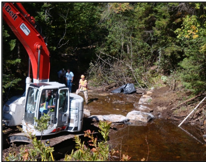
Figure 5.18 Wildlife Friendly Culvert Replacement. A cooperative agency effort (APA, DEC and USFWS) which provided a wildlife friendly culvert replacement on Rte. 28N near Long Lake. The solution included baffles in culvert lining and a stream grade retainer (large stones) to raise water levels.
