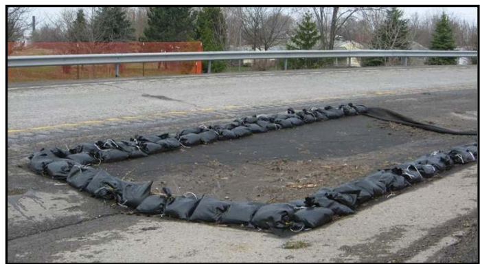
Figure 4.8 Vehicle cleaning station.
