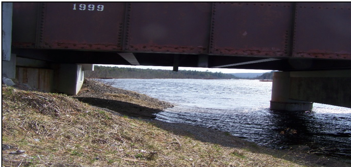
Figure 5.16 Bridge Spans with Upland. Provides greater habitat connectivity.
