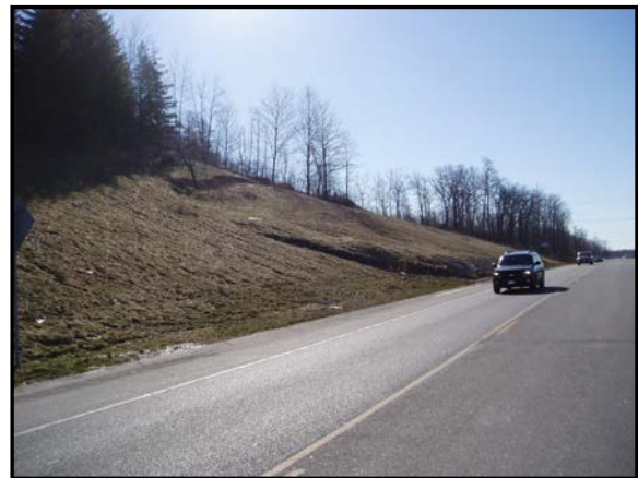
Figure 4.4 Example of slope failure from DOT HDM Chapter 9
