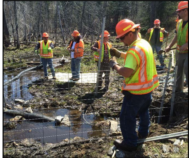
Figure 5.25 Beaver Deceiver. A deep water fence (or “Beaver Deceiver”) was installed as part of this DOT training.
