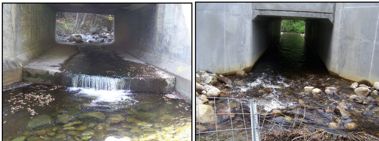
Figure 5.17 Precast Concrete Box Culvert. A box culvert that presents a barrier to wildlife (left), compared to a box culvert that allows for habitat connectivity, by including a natural bottom and placed below stream grade (right).
