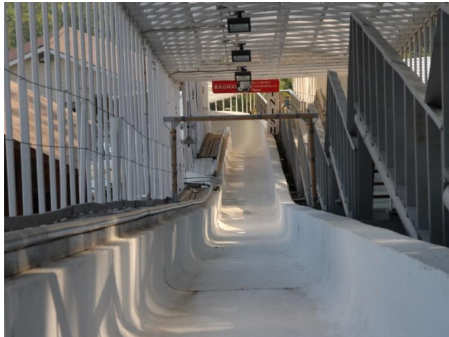
Forward Throw Metal Halide Under Tarp Roof System, No Sidewalls
