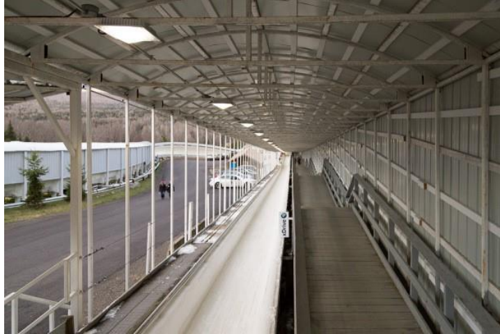
Tin Covered Track with Upgraded, Downward Focused Lighting
