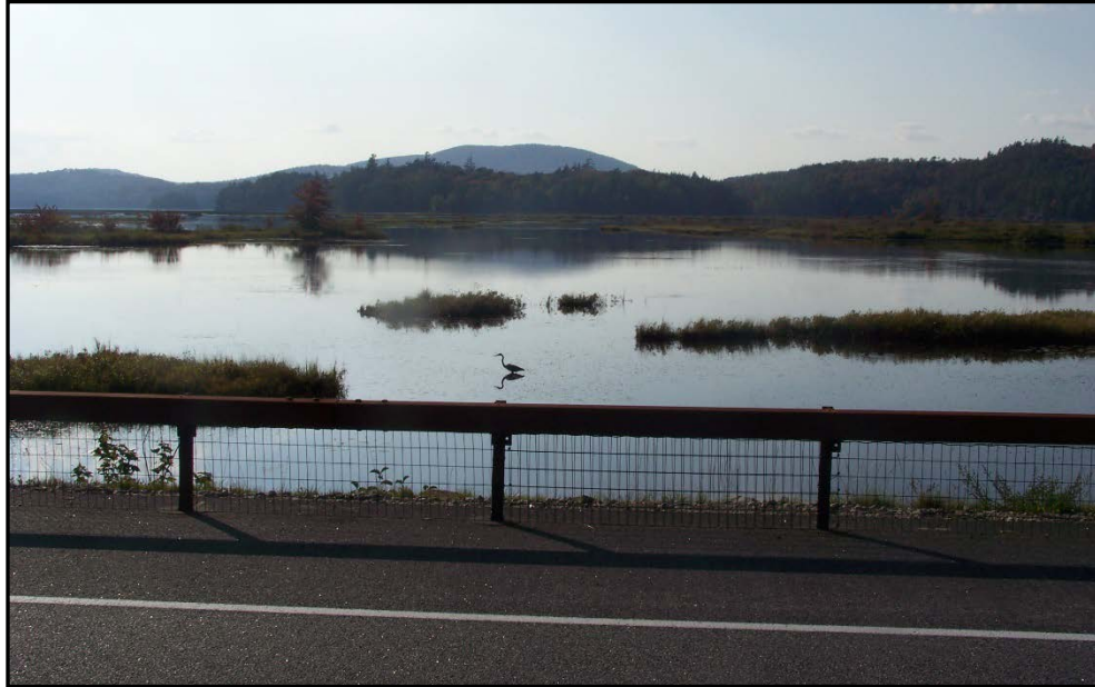
Figure 5.14 Turtle Barrier Fencing. Used to redirect migrating turtles away from road and to safe turtle passage.
