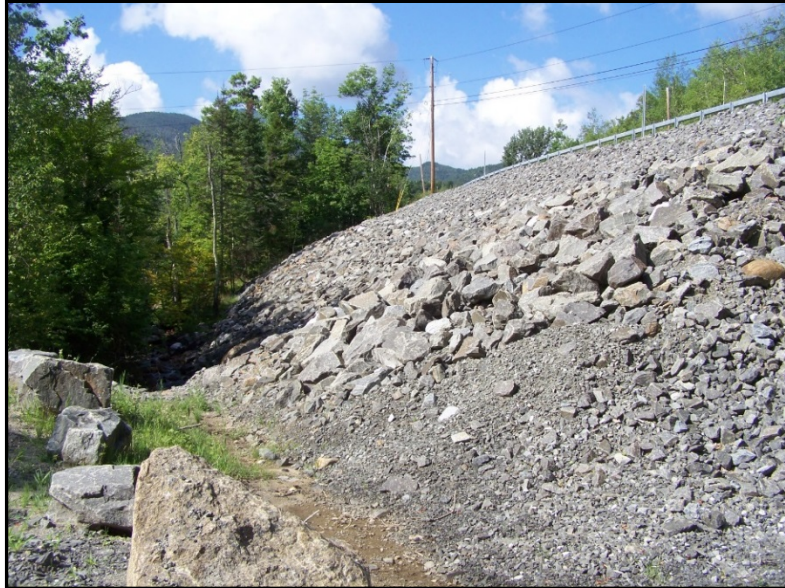
Figure 4.5 Stone slope treatments. Stone slope treatments are a standard practice for slope stabilization, but may not suit the visual context of the Adirondack Park.
